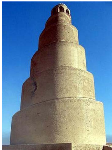
Figure 5. Damage caused to the al-Mutawakkiliyya mosque by a rocket propelled grenade xxxiii
